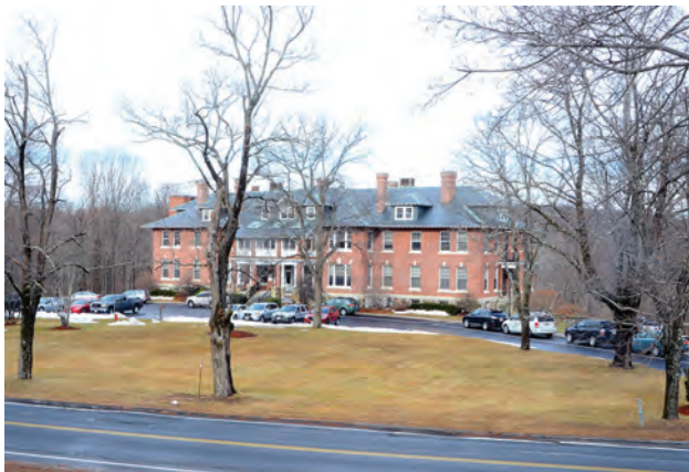
School Green: Jean Mayer Administration Building
