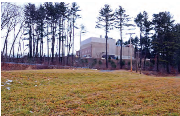
Phase II: View North to Phase I and NE-RBL
