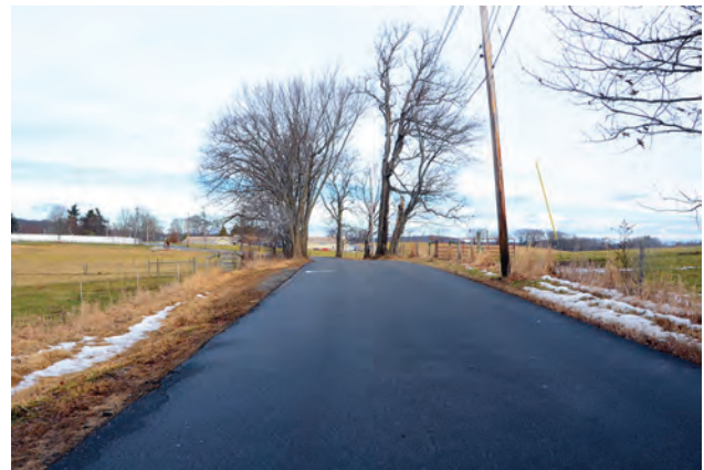
Willard Street: View to North
