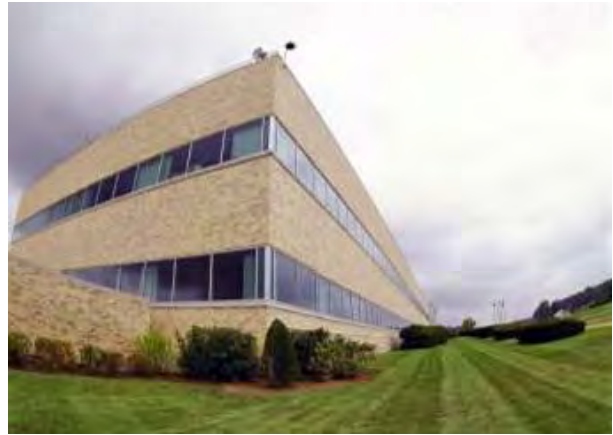
Exterior Shot of Front of Building
