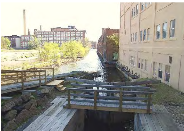
Canal Access and Restored Lock
