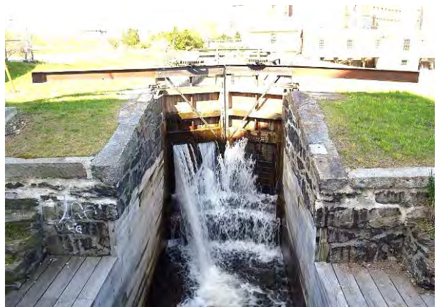
Restored Canal Lock
