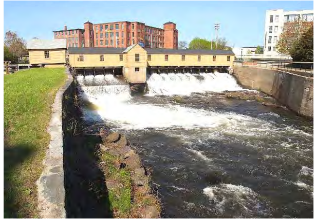
Restored Canal Bridge Structure
