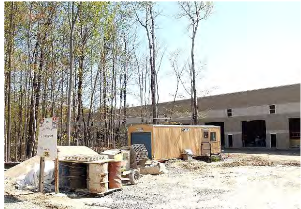
Construction of Spec Building
