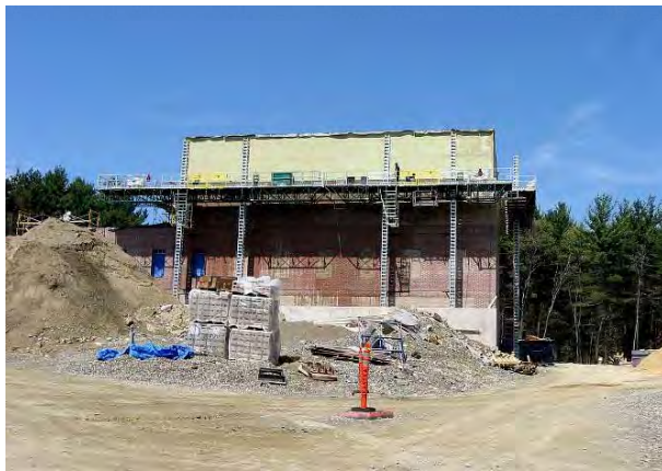
Construction of Disease Research Bldg Across From Site
