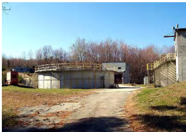
Water Facility Near Border of Gravel Pit Site
