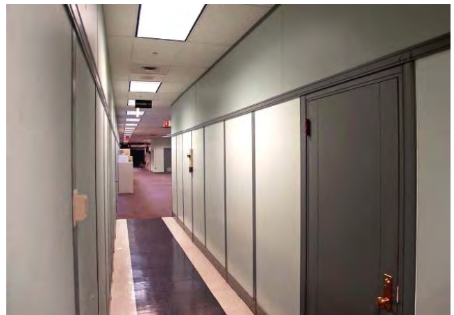
Example of Self-Contained Modular Office Spaces
