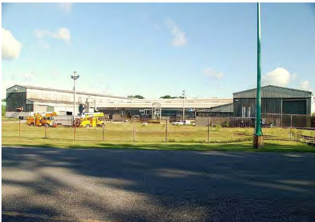
Rear of Manufacturing Building
