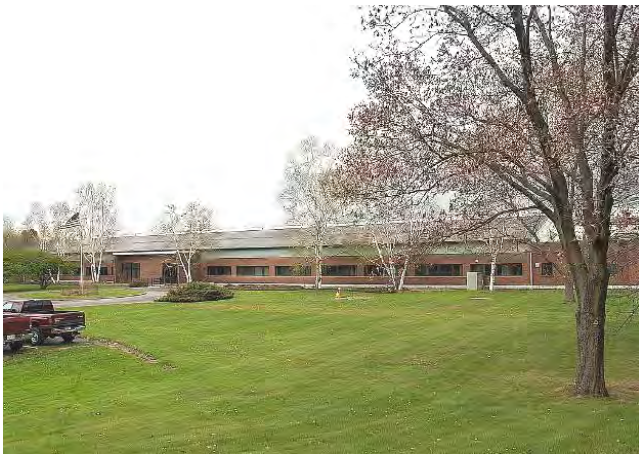
Front of Building and Main Office Entrance
