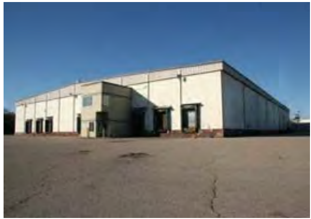
View of Warehouse Loading Docks
